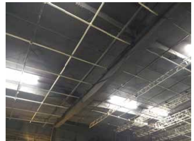
MEGA BEAM SEPARATING GRIDS
